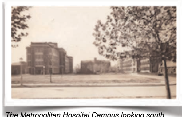
The Metropolitan Hospital Campus looking south. The Octagon building is on the right, its familiar dome hidden by the tree. Photo credit: RIHS archives.
