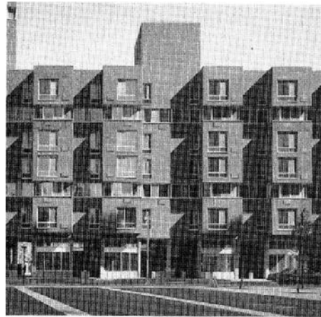
Eastwood's outcropped façade and textured bricks created light, shadow and visual interest. Photo credit: David Hirsch.
