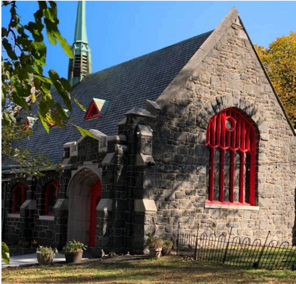
From Episcopal Chapel of the Holy Spirit to Dayspring Church to a proposed new chapter in its life, the little stone church on the northwest side of Roosevelt Island has had its ups and downs (see p. 9). Photo credit: Bobbie Slonevsky.
