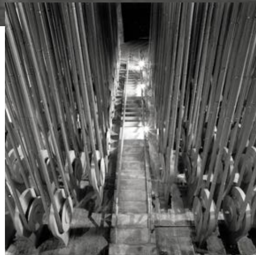
Cable strands, eyebar, Staten Island anchorage.
