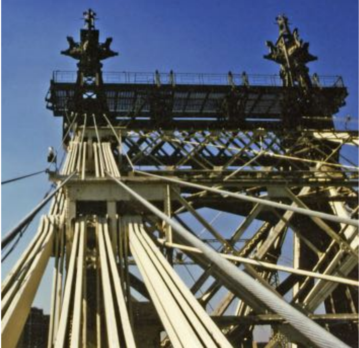
Recognize it? It's a tower of the Queensboro Bridge (see "Getting Here! Bridge(s) over Turbid Waters," p. 2) photographed by bridge-climber/photographer Dave Frieder (see "The Magnificent Bridges of New York City," p. 9). Note the innovative eyebars used instead of cable. Until 1960 the decorative finials held flag masts, but they rusted so badly they were removed. Now the top of the finials are outfitted with aviation beacons.
