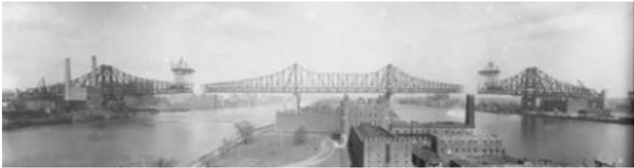
Cantilever Construction: Cantilevers are structures that project horizontally into space, supported on only one end (like a diving board). Cantilever bridges are economical to build, they are stronger than suspension bridges, and they allow for long spans and wide clearances under the span. The Queensboro Bridge is an example of double cantilever construction: the Manhattan and Roosevelt Island cantilevers meet and pass over the west channel of the East River, while the Roosevelt Island and Queens cantilevers cross the east channel. There is a smaller truss connecting the two island piers. This photo shows traveling cranes ready to position the final sections of the roadway. Photo: New-York Historical Society Collection.
