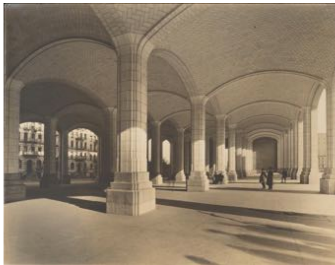
Vaulted Arches with Guastavino Tile: Looking east from Second Avenue, this space under the Manhattan approach housed a vibrant market from 1914 until the 1930s. After being demoted to a grimy storage area for decades, it was restored to its former splendor in 1999 as the Bridge Market. Photo: Museum of the City of New York.
