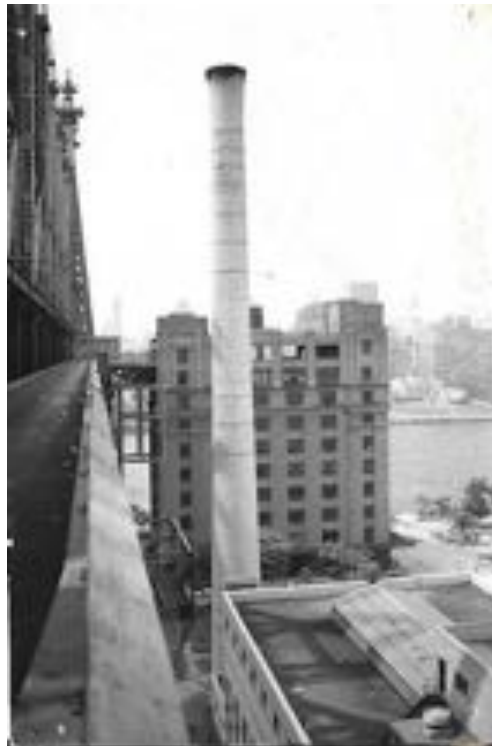
The Elevator Storehouse: Looking west, the building on the north side of the bridge provided convenient access to Blackwell's Island day and night. Those traveling east on the south side of the bridge, stepped into a passageway that crossed under the roadbed to the north-side entrance to the building. Photo: The Eleanor Schetlin Collection at the RIHS.
