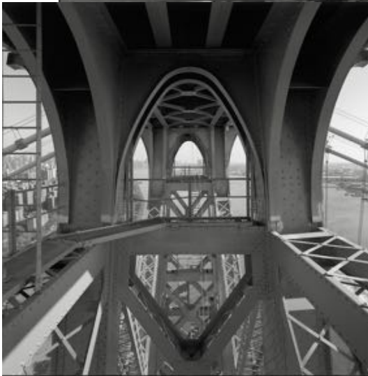
View from service walkway through Manhattan tower.
