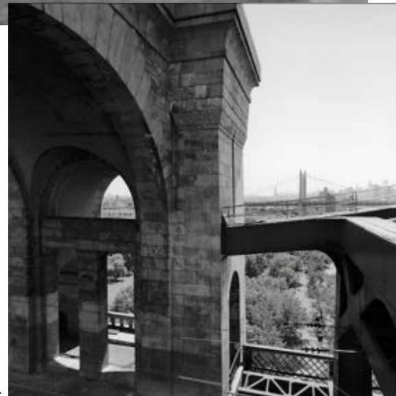
View of stonework detail from upper chord.
