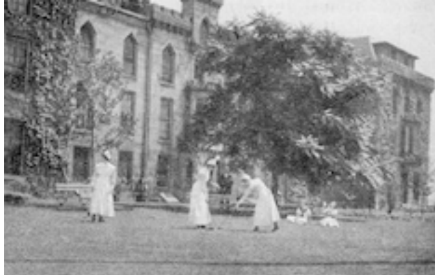
An additional wing was added onto either end of the hospital (see right) once it became a nursing school. Photo credit: NYC Department of Public Welfare.
