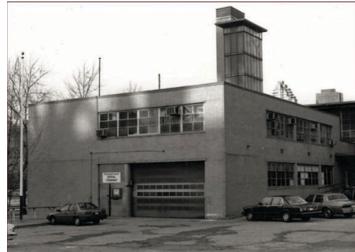
A new firehouse was built in 1949 on a site just north of the 59th Street Bridge near today's tram station. The unique brick and glass hose-drying tower is visible at the back.
