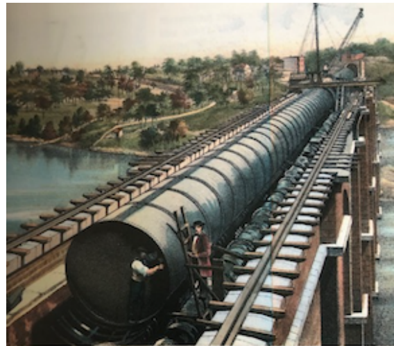
Croton water crossed the Harlem River in two iron pipes atop the High Bridge. Credit: The Historical Atlas of New York City.
