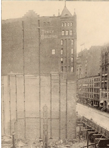
The Tower Building at 50–52 Broadway was the first building in New York City to use a steel skeleton. It was completed in 1889 and was 11 stories high. Image: https://en.wikipedia.org/wiki/Tower_Building .
